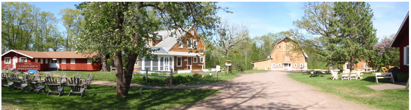
L to R: Cross Dorm, Farmhouse Office, Barn Dining Hall, Program Garage, Library
